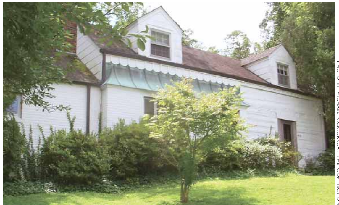
Birchwood at 4756 26 th Street, North.
