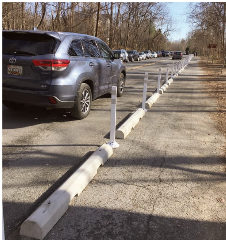
Temporary barriers were put in place on the south side of MacArthur Boulevard between Anglers Inn and Brickyard Road in late November. The barriers separate bicyclists and pedestrians from traffic and prevent parking along that side of MacArthur.
