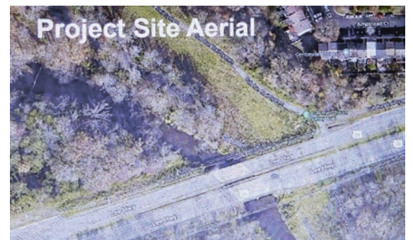
A view of where the bridge work is happening along northbound Route 29 over Cub Run in Centreville.
