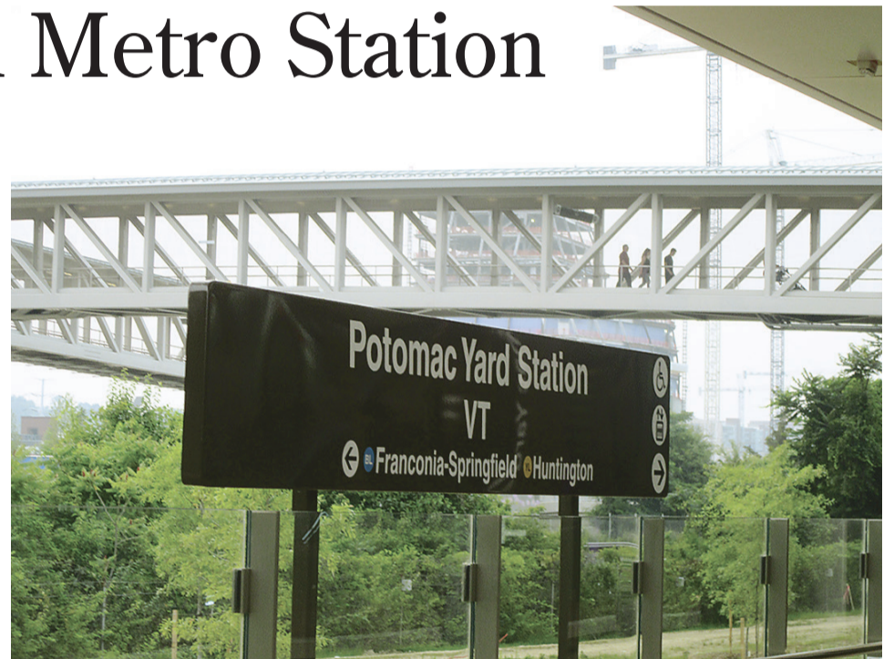
An aboveground covered walkway connects the two entrances/exits of the new Potomac Yard Metro station.
