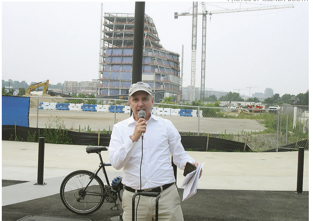
Stewart Schwartz took the June 6 group to the station's deck. The building under construction is the first of three planned for the new Virginia Tech campus.
