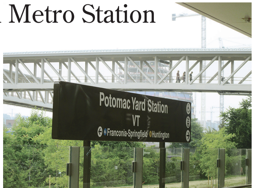
An aboveground covered walkway connects the two entrances/exits of the new Potomac Yard Metro station.
