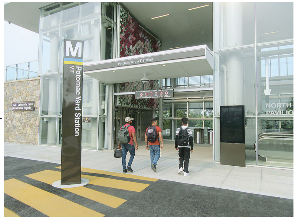
The new Potomac Yard Metro station's north entrance
