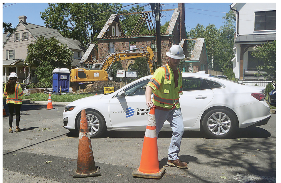
Dominion Power is checking out downed power lines in the Clarendon area. Tens of thousands of people were without power in Arlington, some until Tuesday.
