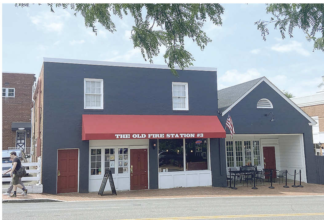
Across from Old Town Hall, Old Firestation #3 is open seven days/week.
