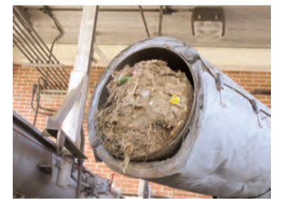
Compacted materials removed at the Noman Cole plant from incoming water, including plastic, wipes, fabrics and fast food debris.
