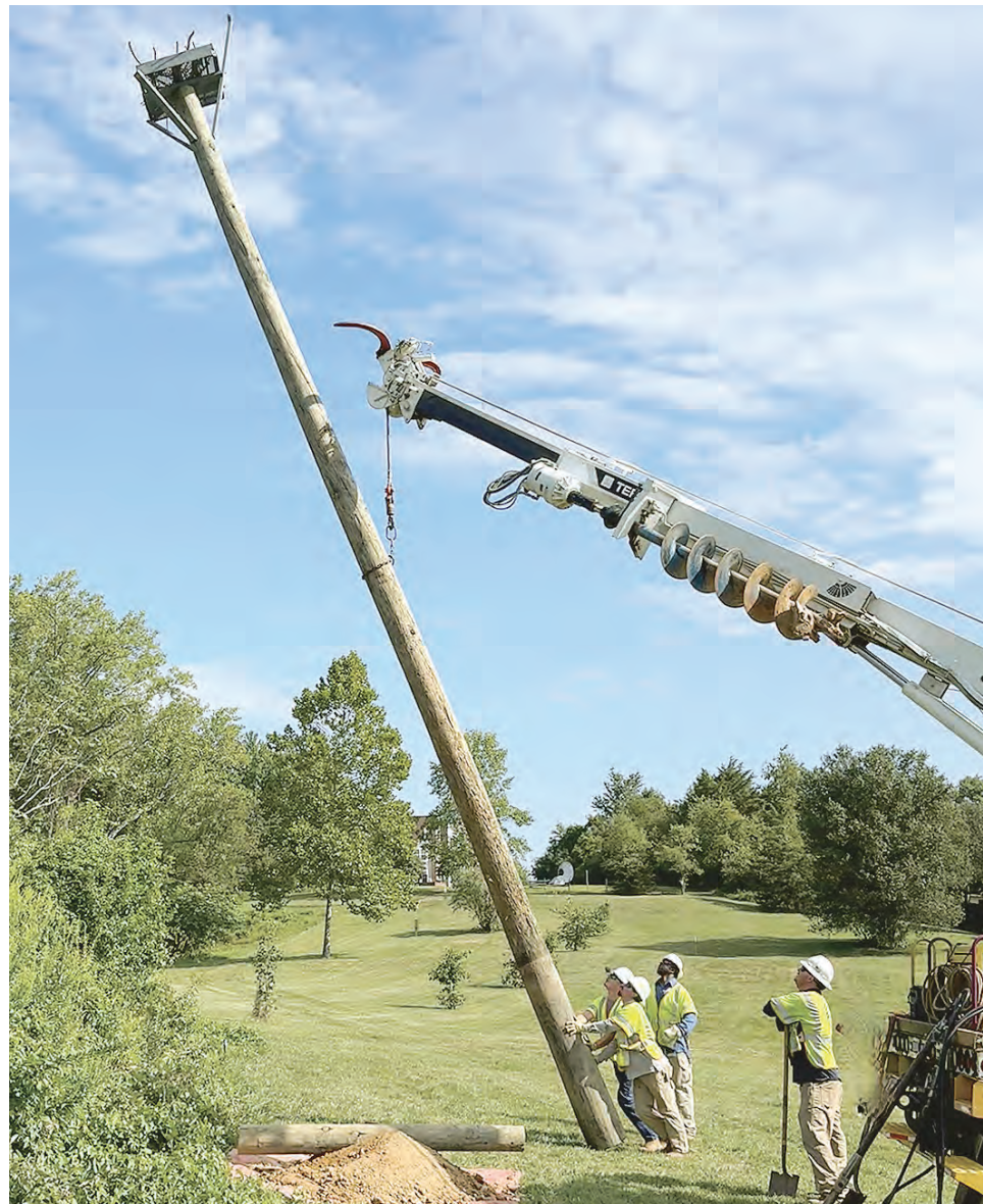
With auger retracted, the derrick with pole guides and winch maneuver the pole
