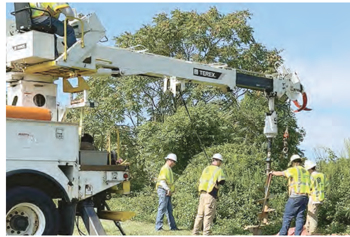
Ryce Zink operates auger to create deep hole to accommodate platform pole
