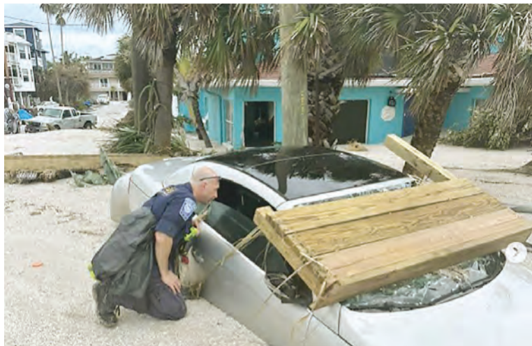
On Saturday, VA-TF1 members conducted primary searches on buildings in Treasure Island, Fla., checking for damage and any victims needing assistance. The team has been reassigned north and is traveling to the Carolinas to provide additional assistance.
