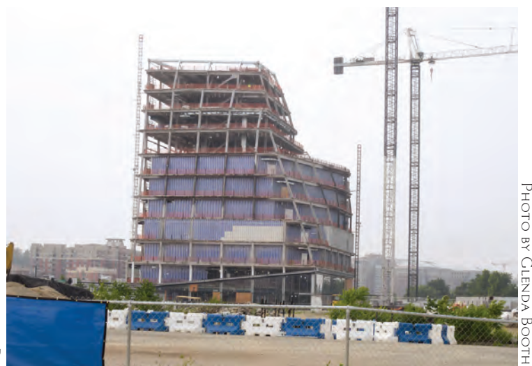
The Virginia Tech Innovation Campus building under construction in 2023.
