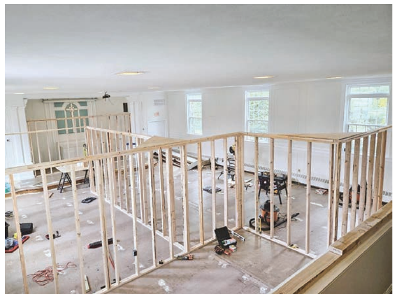
It didn't take long to get the project going.
