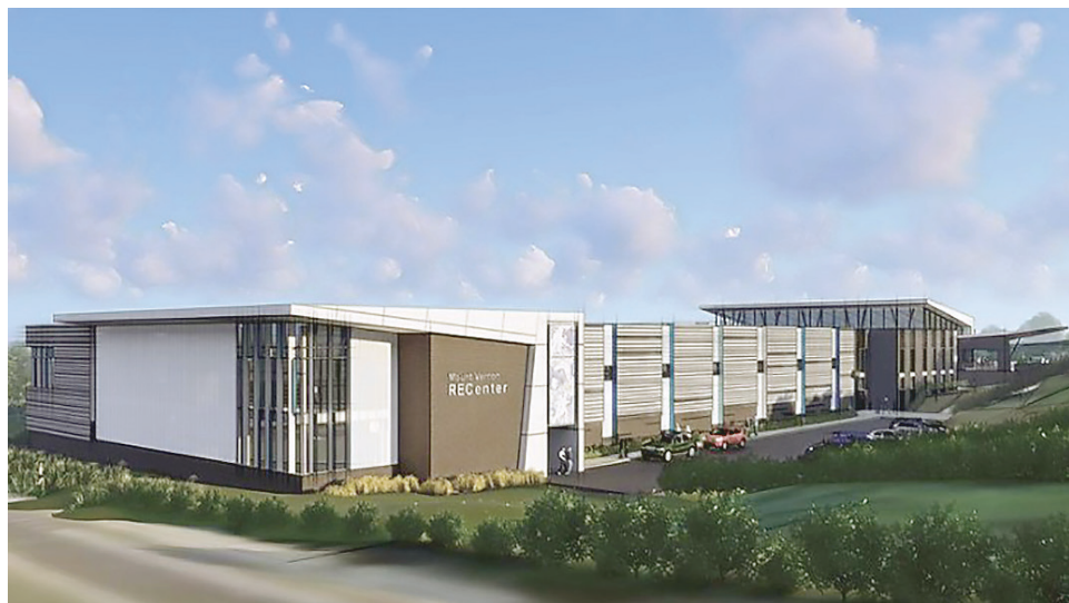
The renovated rec center in Mount Vernon will be a big addition in 2025.
