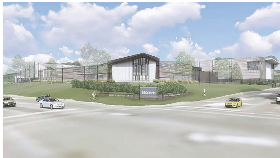
A two-story fitness center is included with the renovated rec center in Mount Vernon.
