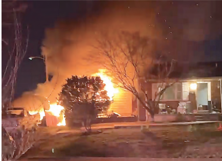
PHOTOS COURTESY OF FAIRFAX CITY FIRE DEPT. Flames greeted first-arriving units when they reached the home.
