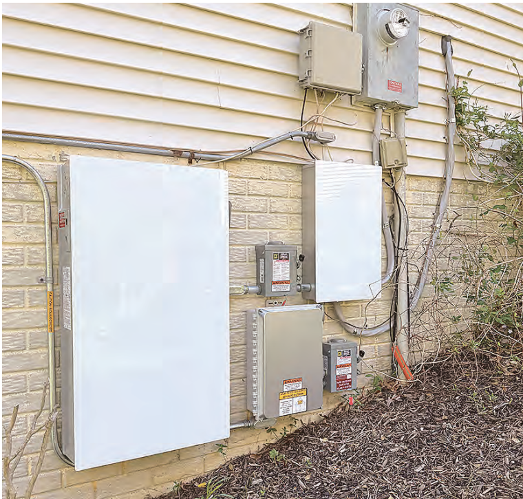
System control panels can be mounted outside, or in a garage with recommended bollard protection
