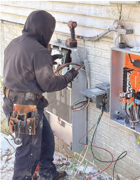
An installer electrician connects a back-up battery adjacent to the installed solar panel controller
