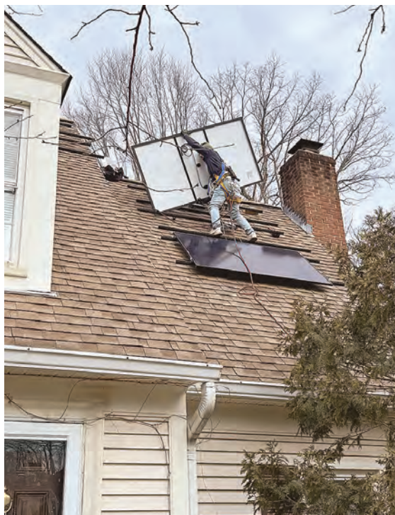
Solar panels have become smaller, lighter, and more efficient, easily maneuvered onto racking rail equipment
