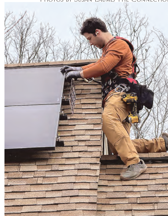
Installer adds a recommended "critter guard" to prevent small mammals from chewing wires, or birds from nesting
