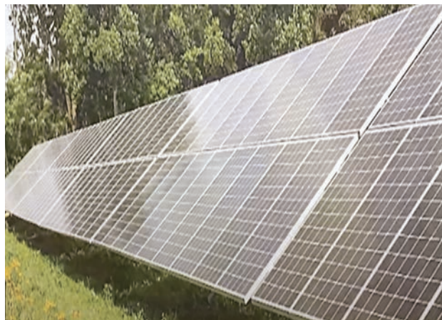
Lorton's solar array field will consist of 12,000 panels covering 37 acres of closed landfill.
